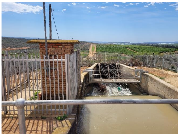
Figure 15: Existing siphon off-taking from Kirkwood Primary Canal similar to the proposed siphon infrastructure
